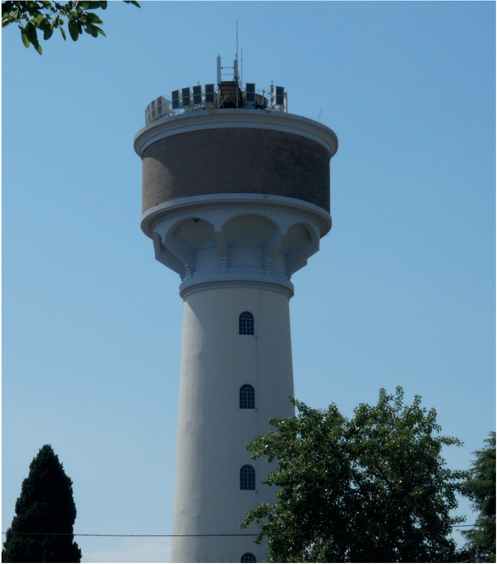
Fig. 2. The water tower
