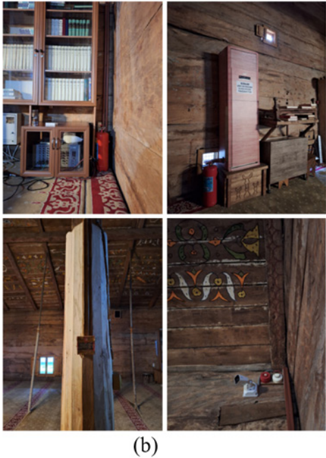
Fig. 4. Escape distances in the plan of a historical wooden mosque (a) and portable fire extinguishers and fire warning-alarm and smoke detection systems (by author)
