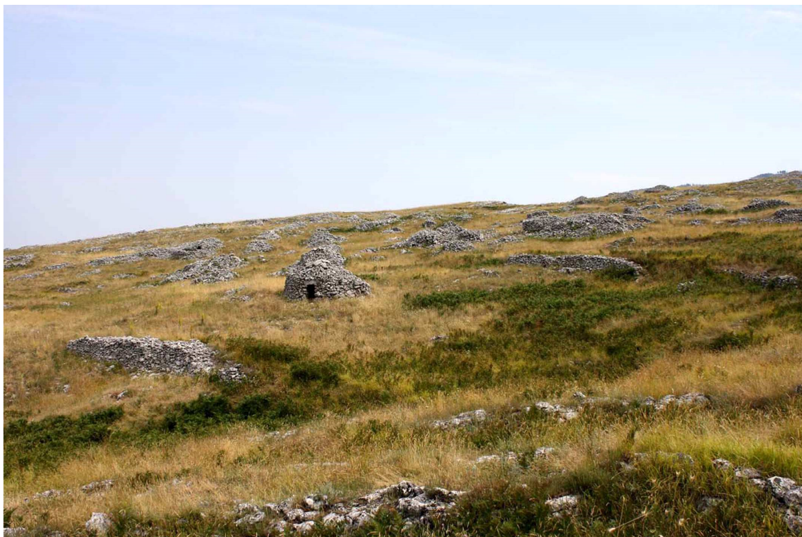
Fig. 7. Agro-pastoral landscape in the area of Roccamorice (PE). The most remarkable features of this landscape are the dry-stone masonry, the tholos huts used by both shepherds and farmers, and the piles of stones removed from the fields.
